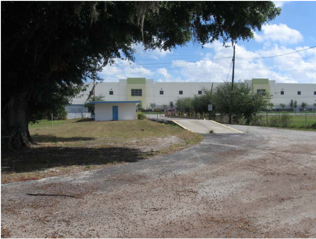
FROM WAREHOUSE-LOOKING AT ENTRANCE
