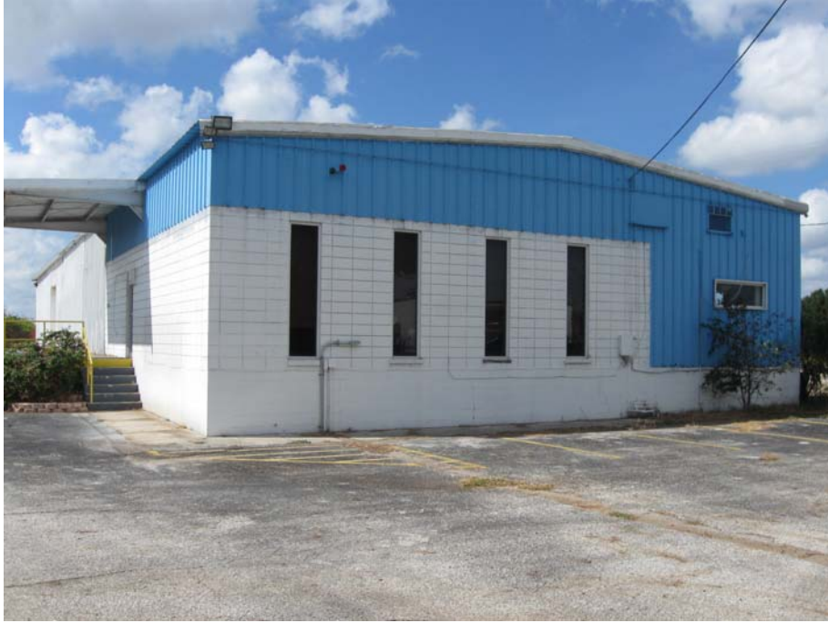
WAREHOUSE OFFICE ENTRANCE
