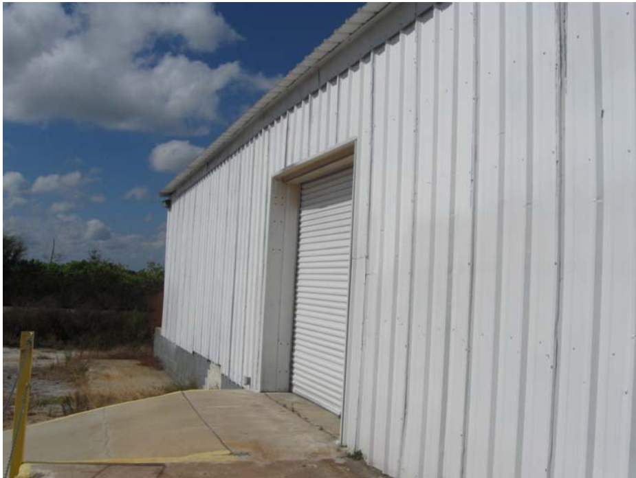
WAREHOUSE DOCK AND RAMP
